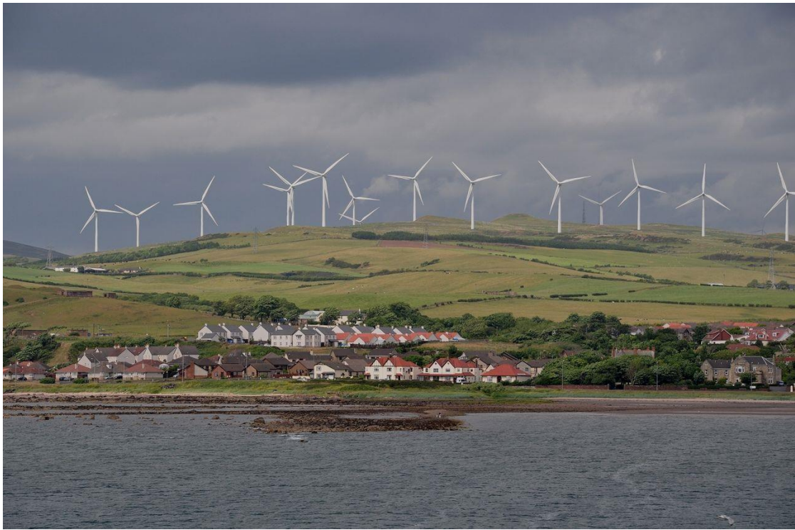
Wind farm above Ardrossan
