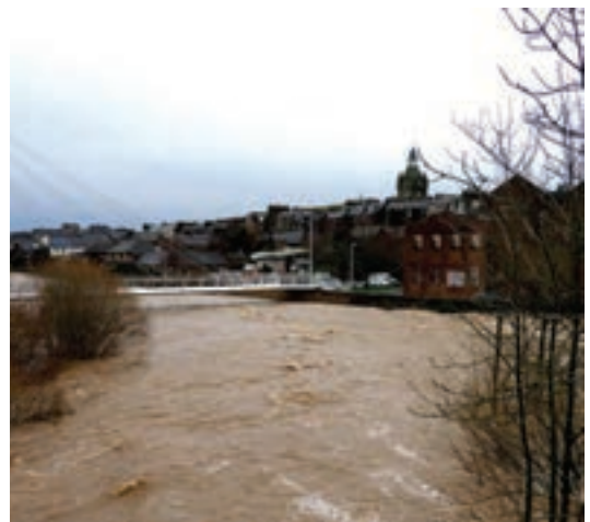
Flooding at Hawick, January 2017 © Duncan Bryden
